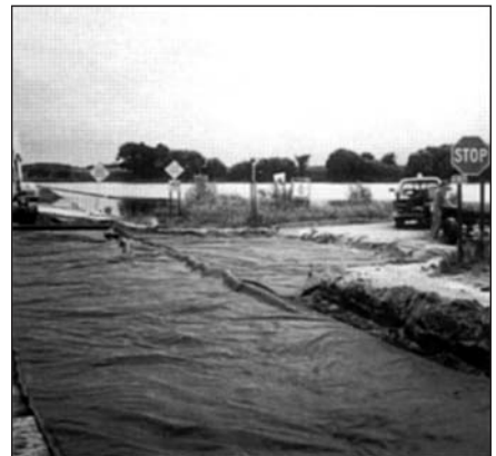
Mirafi® 600X used for stabilization in roadway repair
